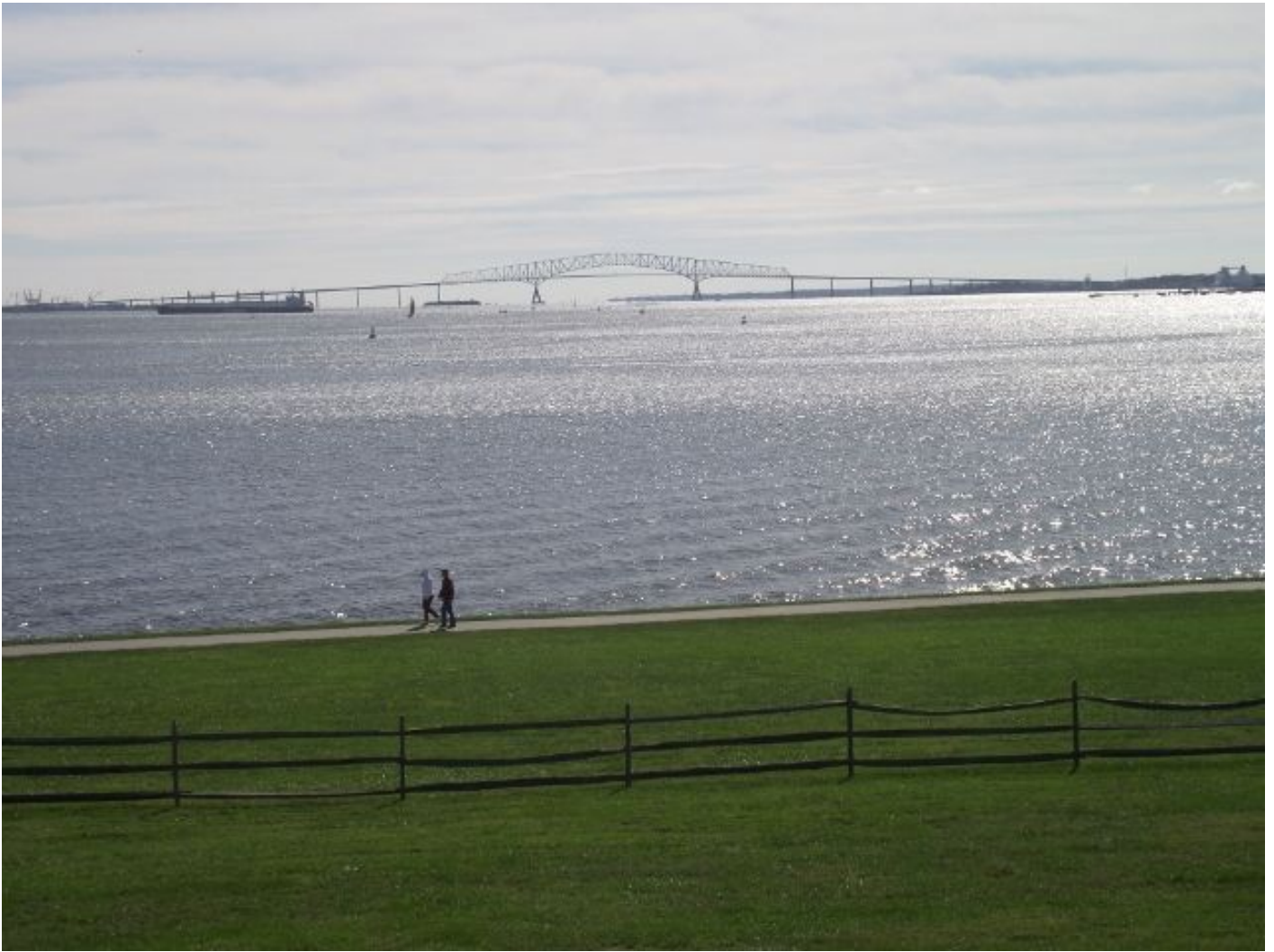
The Francis Scott Key Bridge is two miles from Ft. McHenry. The British bombardment ships in 1814 remained in the area of the present-day bridge to stay beyond the range of the cannons in the fort.
